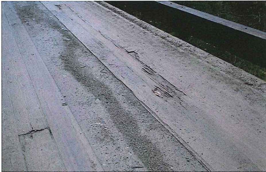
CK2139 Deck condition
