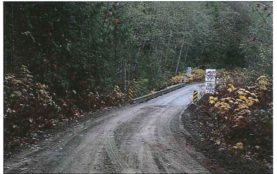
CK2139 Approach Right Bank
