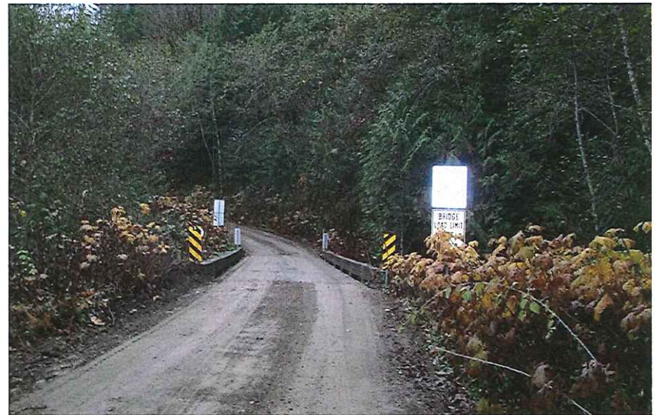
CK2139 Approach Left Bank
