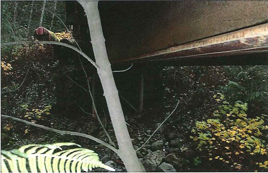
CK2139 Abutment Left Bank
