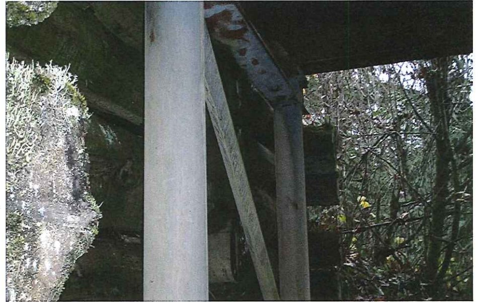
CK2139 Abutment Left Bank #2
