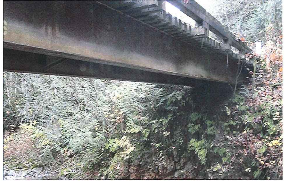
CK2139 Crossing Upstream
